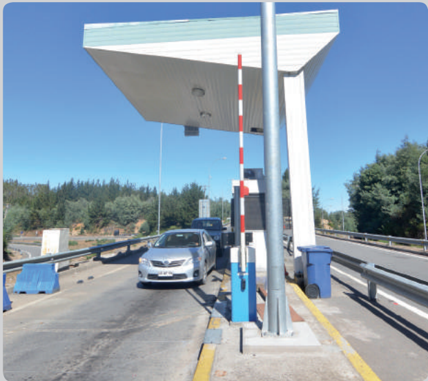
Plaza de peajes, Ramal Rafael / Toll Plaza, Rafael Branch
